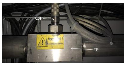
For **installation of CSF** the customer needs a **threaded installation bush**. Some customers additionally use a locking set (this is a simple chain) for security reasons. 对于安装CSF,客户需要一个螺纹安装衬套。由于安全原因,一些客户还使用了锁集(这是一个简单的链)。
